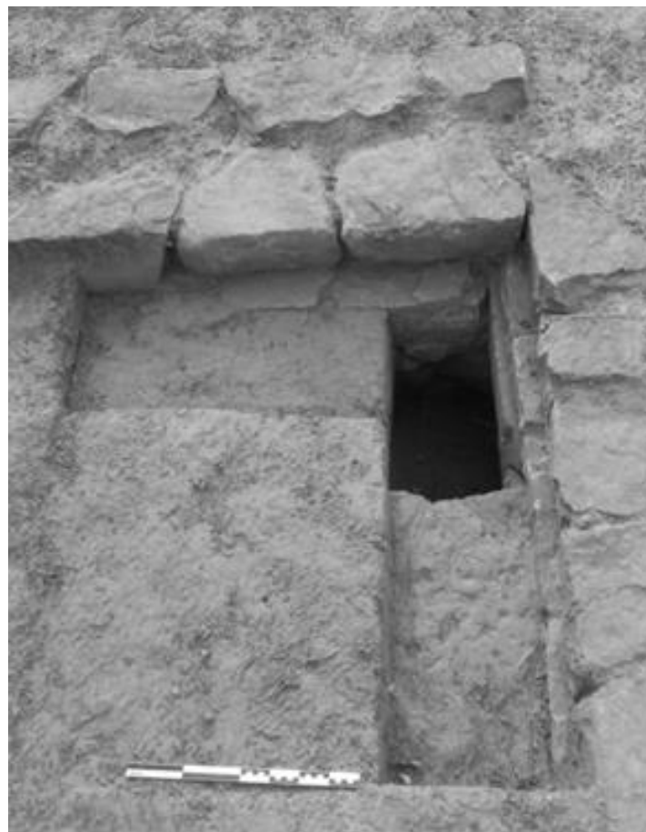
Figure 5. Photograph of the ledge in the stone foundations excavated at the PPH structure.
