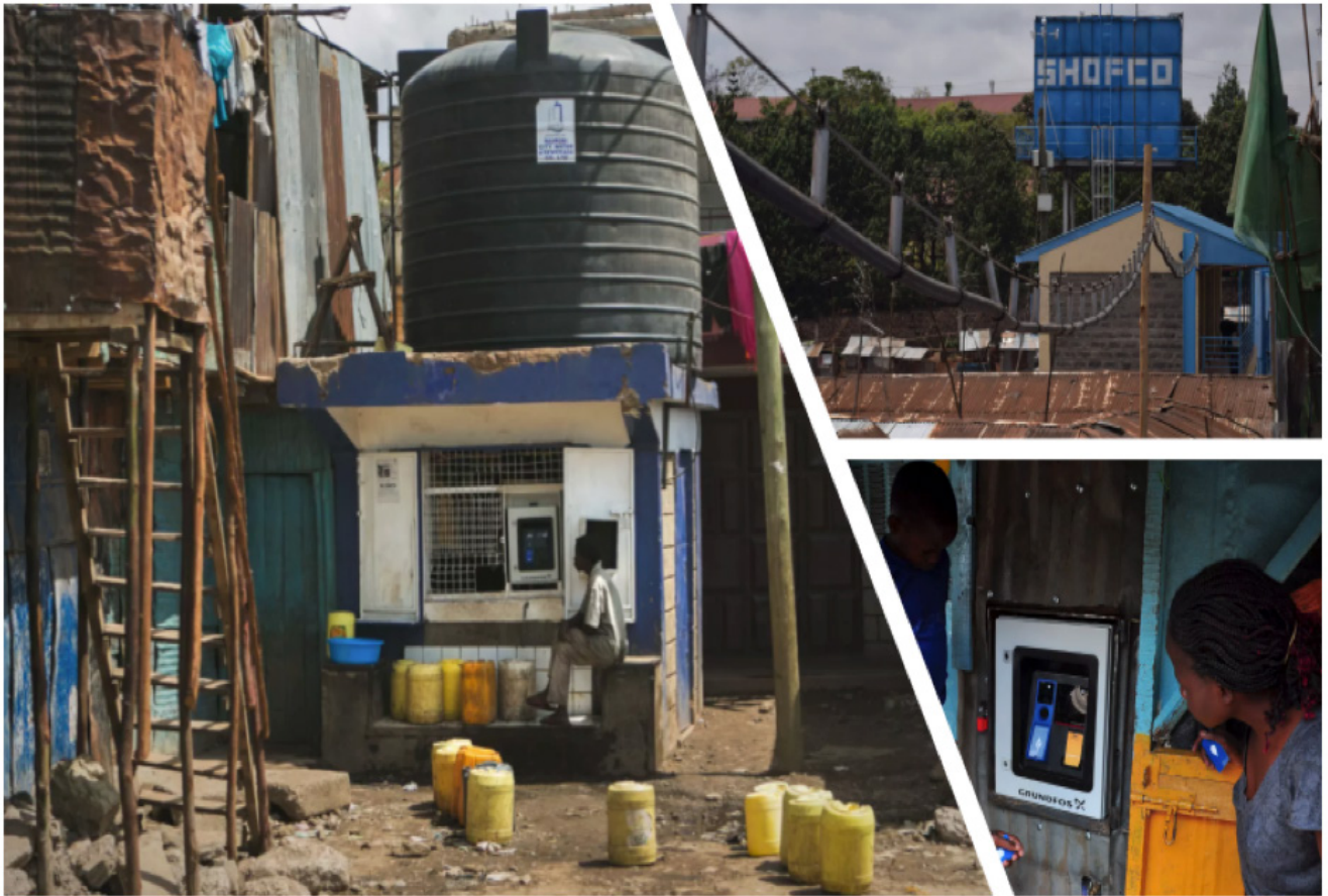
Image 1: Water ATM Vending Machine in Mathare Slum (left) (UNFCC/Chris McMorrow); Aerial water system in Kibera (top right) (Daniel Wesangula); Water ATM in Mathare Slum (bottom right) (Grundofs)
