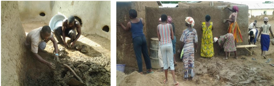
Figure 1: Collaborative wall construction and finishing process
