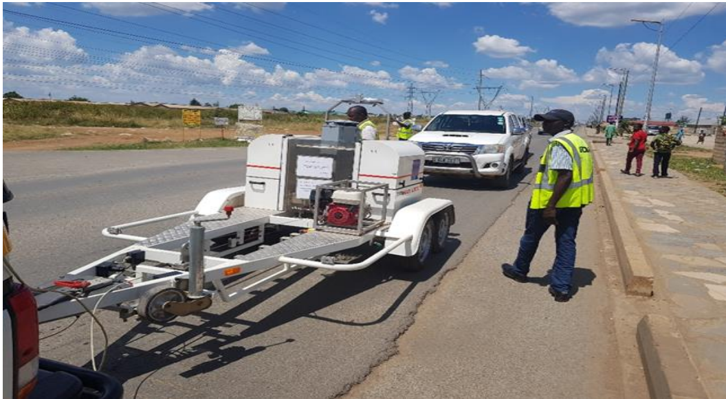
Figure 1. FWD testing ongoing on one of the study road sections
