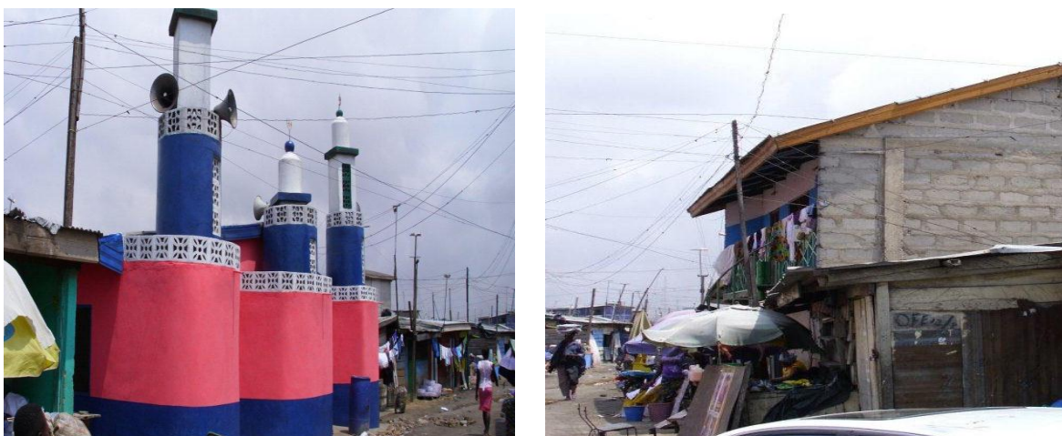
Figure 1: Haphazard and Dangerous Electricity Connections in the Slums
