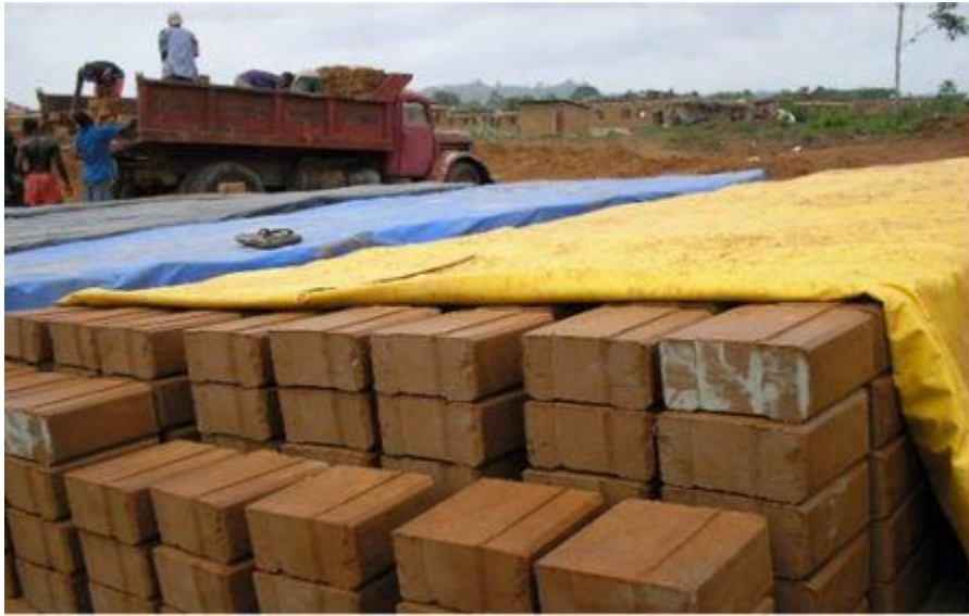
Figure 2: Curing and stacking of interlocking blocks (Source: Researcher's field survey, 2007)
