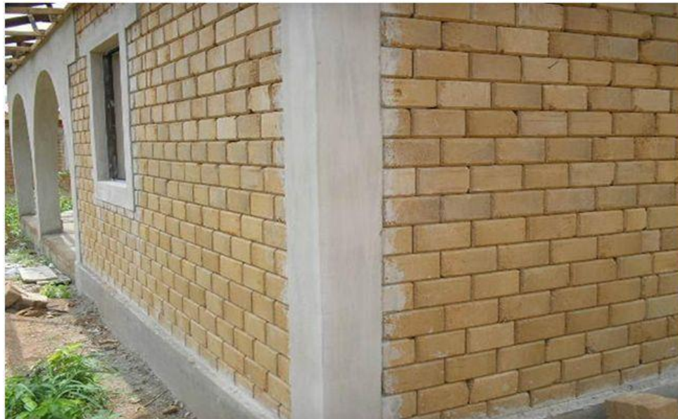
Figure 4: Solid interlocking blocks used for construction of a housing unit at one the selected sites (Source: Field survey, 2010)
