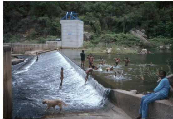
Figure 1b. A dam wall along the Umgeni River between Pietermaritzburg and Durban [Grp 9/19].
